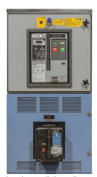
replace the vintage power circuit breaker with new current technology and replaces all the cell structure envelope in which it engages both mechanically and electrically.
