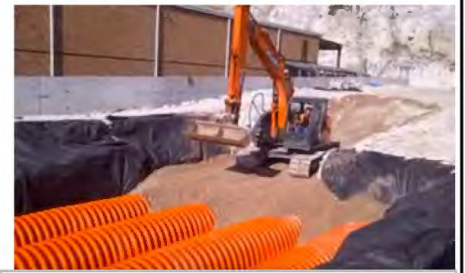
Crushed Washed Stone Cover
