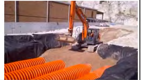
Crushed Washed Stone Cover
