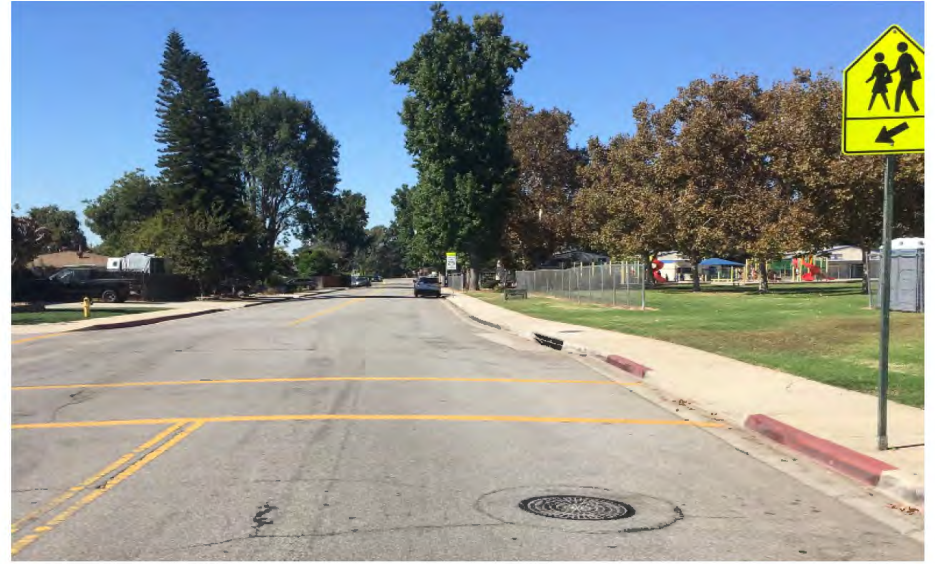
Photo 5 - Secondary Connection Location
