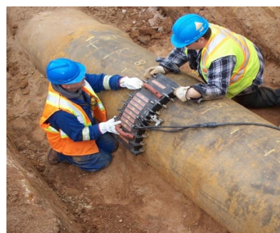
External Condition Assessment Bracelet Probe including Ultrasonic Testing (UT)
