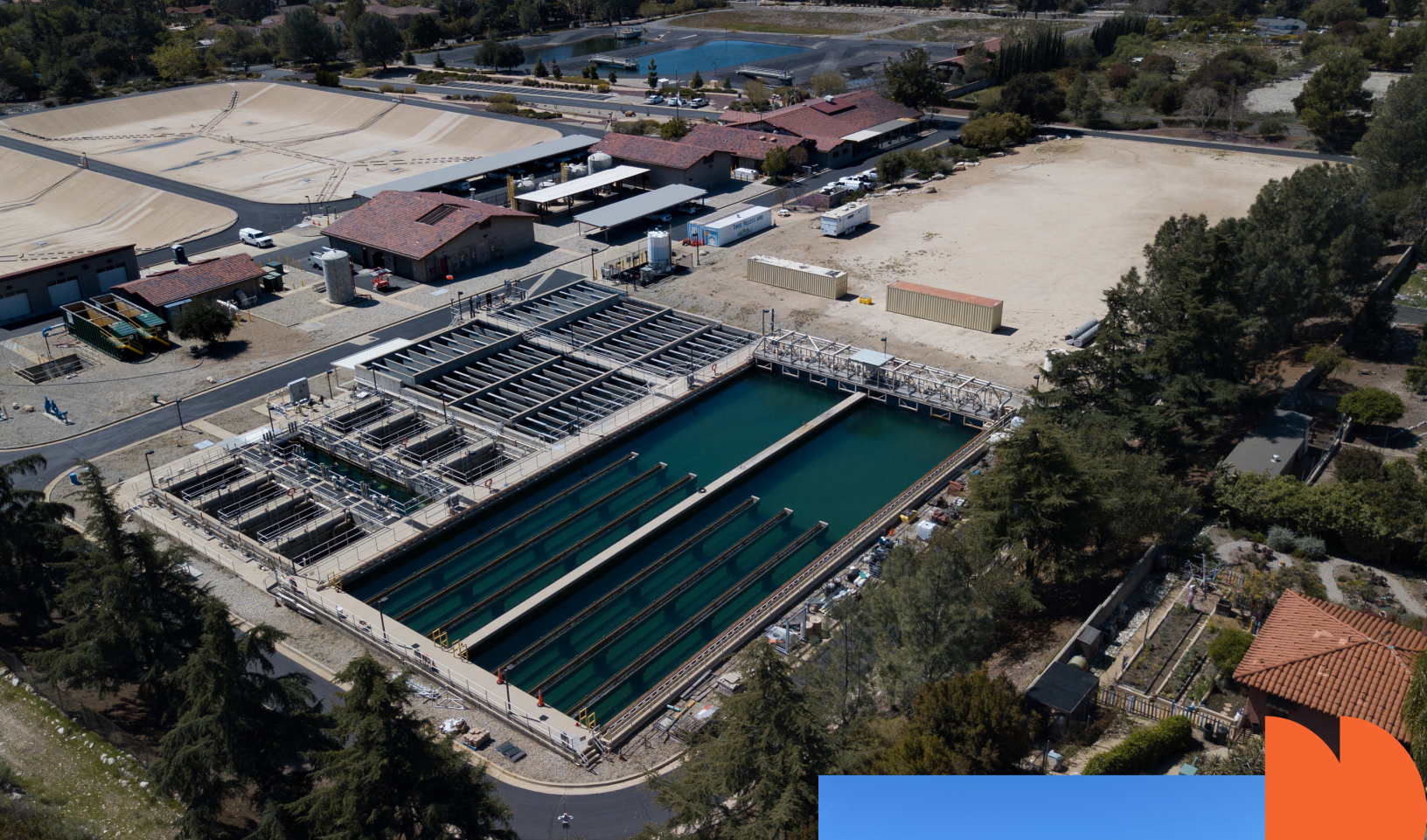
Miramar Treatment Facility pictured above. Three Valleys staff pictured to the right performing annual preventative maintenance.
