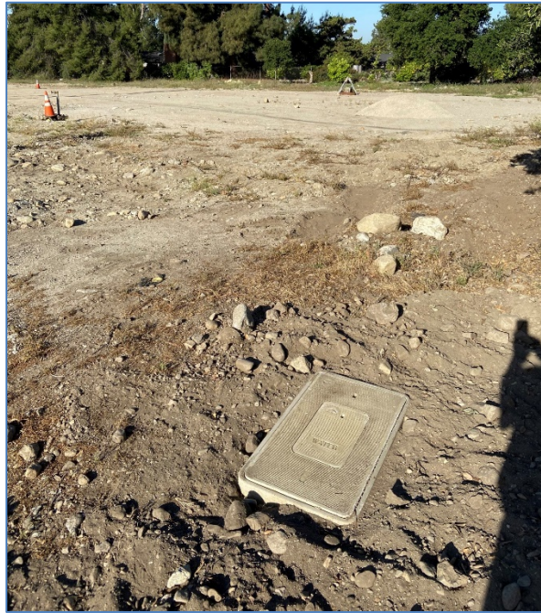
POTABLE WATER METER 1.5-INCH CONNECTION View Looking West on Grand Avenue
