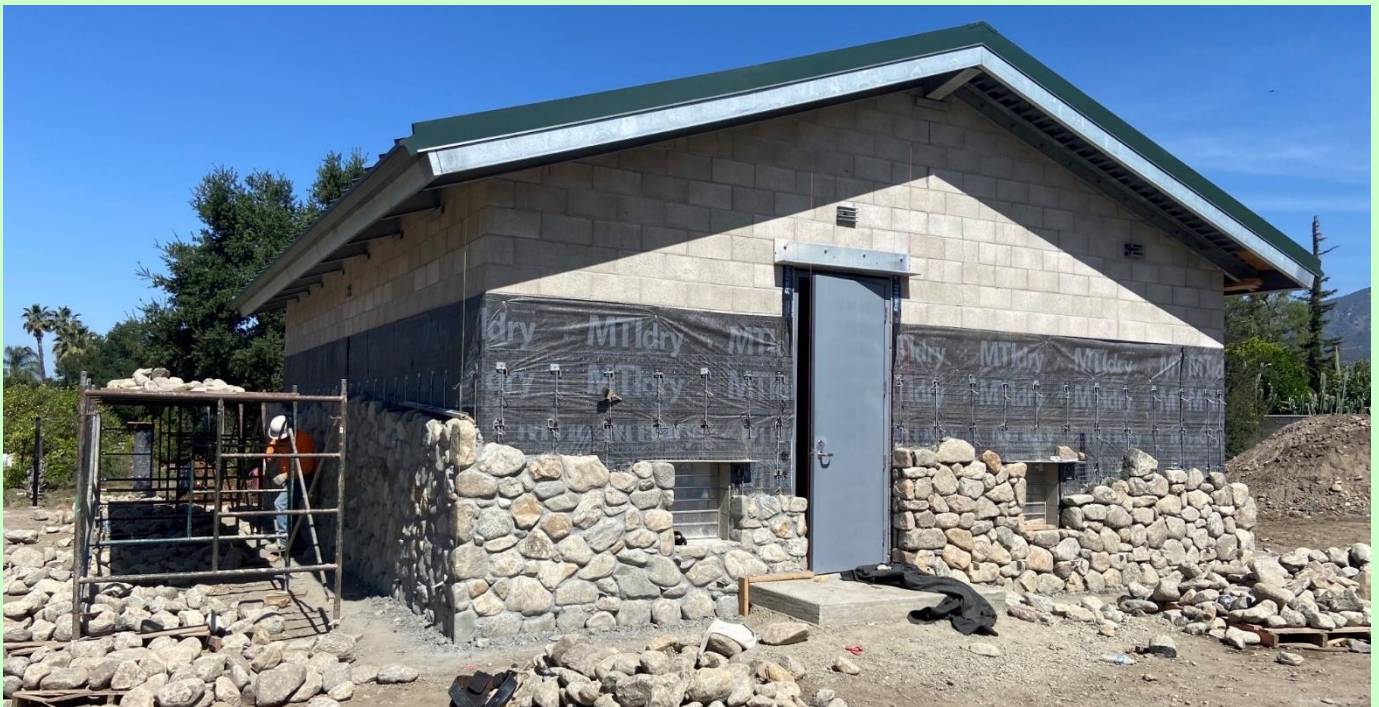
Miragrand Well Enclosure - Field Stone Application to Walls
