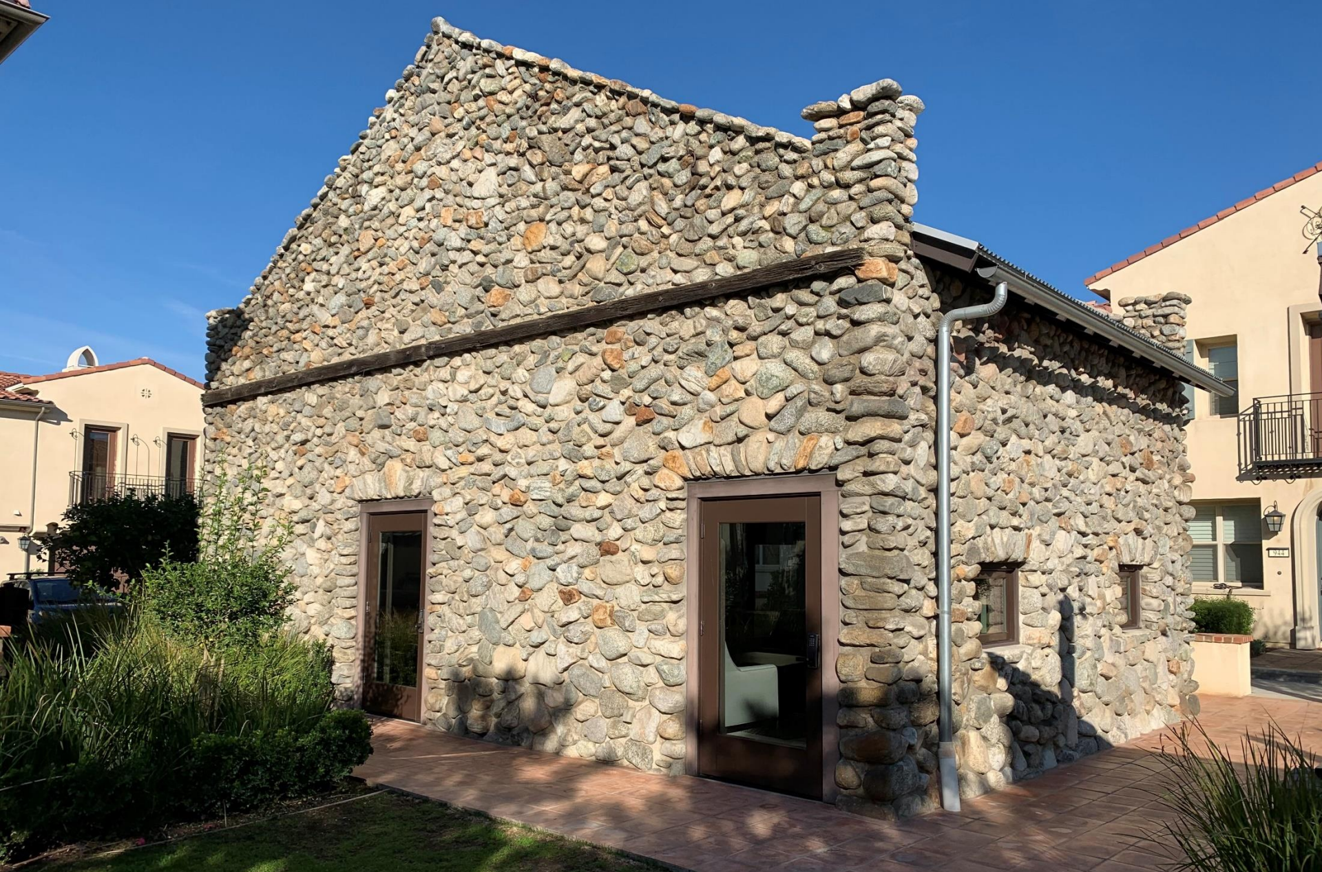
Historic Fieldstone Barn – Baseline & Padua
